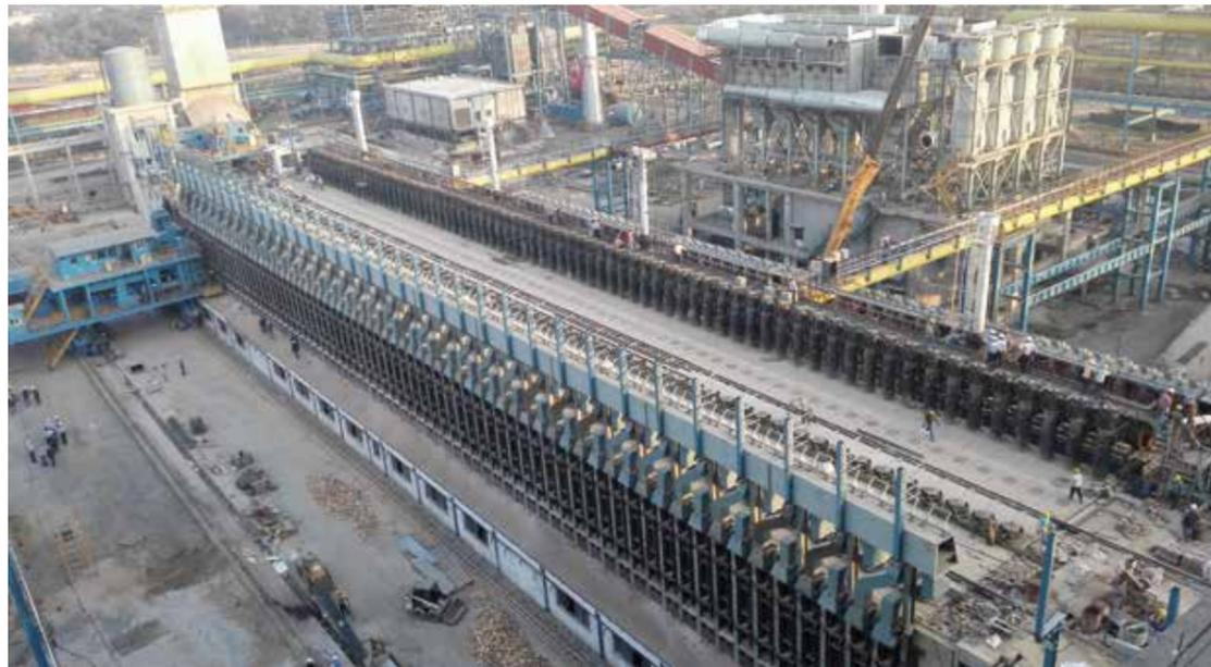
The JSPL coke oven plant, located in Angul, 160km northwest of the capital of Odisha State, will produce 1.9 million tons coke per annum. Sinosteel MECC's layout concept includes 4x72-chamber coke oven batteries, which is 4.3m TJL4350F type stamp-charging featuring twinfuel underjet, combination fired and waste gas recycling, 3-mtpa by-product facility, and 1.1-mtpa coke oven as well as coke quenching to be preserved.
