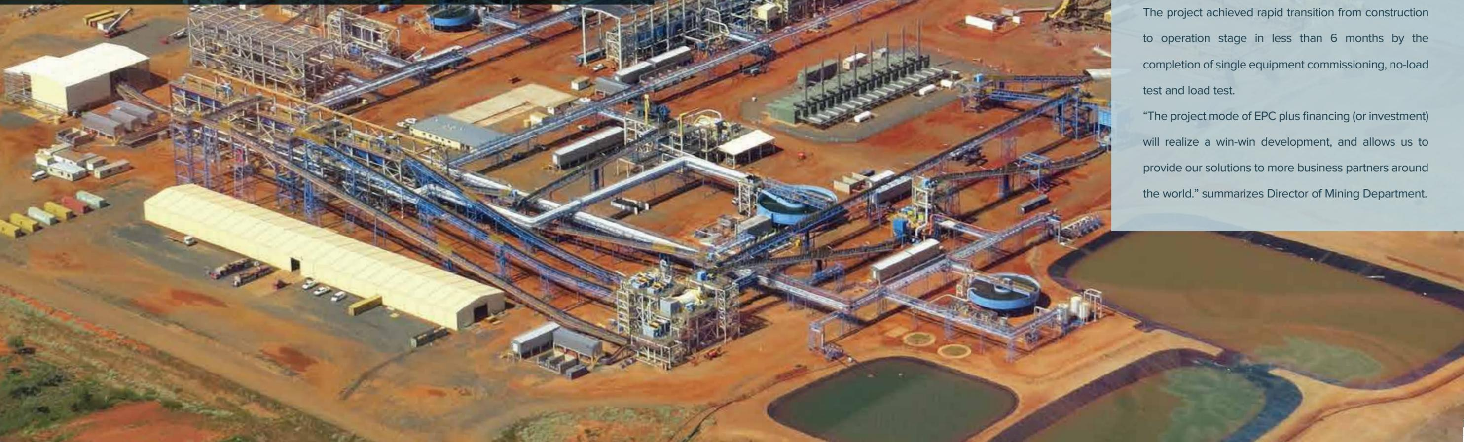
With the application of 3D design, as well as modularization and preassembly for steel structure and pipeline, Sinosteel MECC efficiently reduced the construction difficulties and cost.
