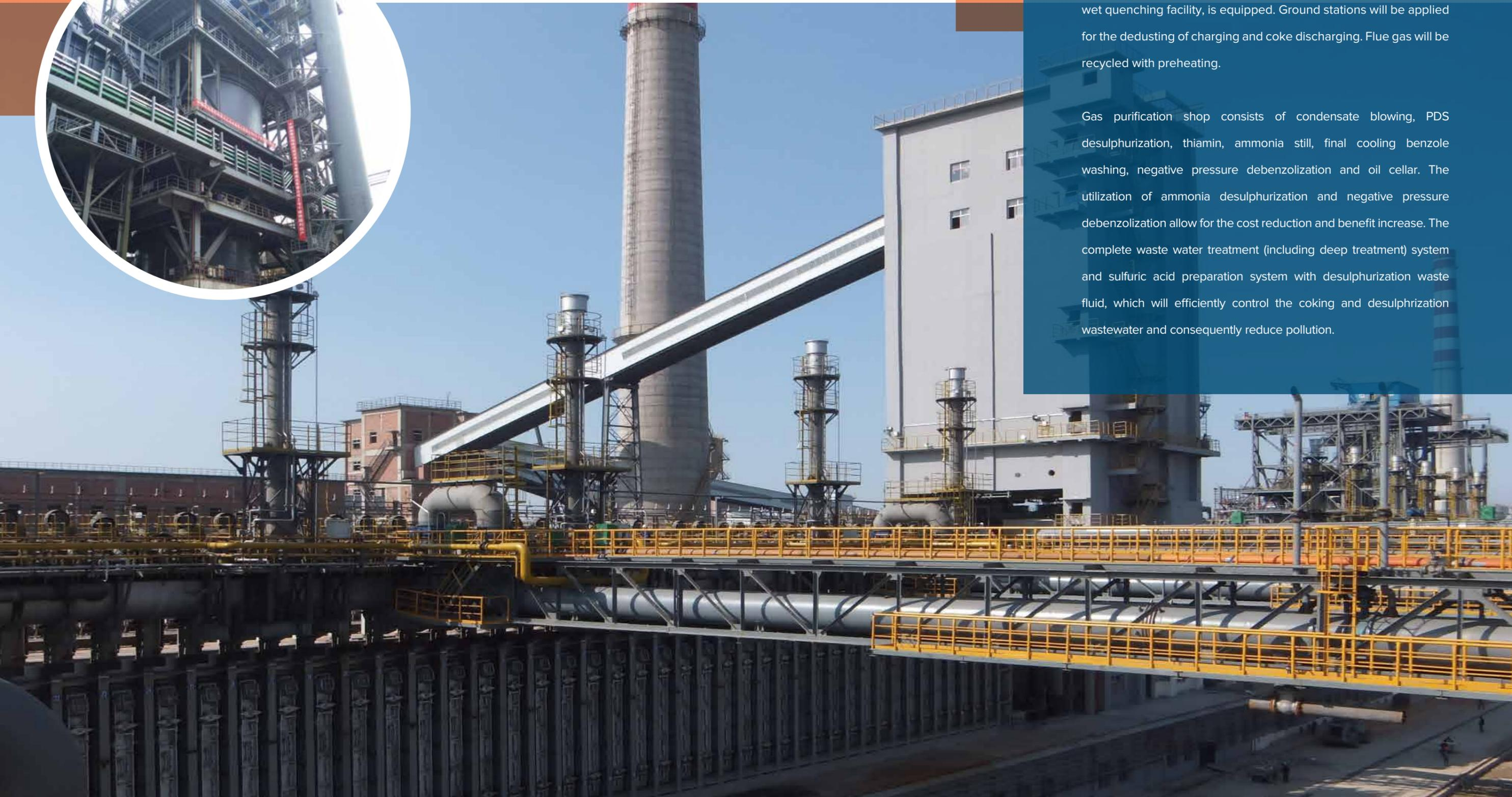
As part of comprehensive energy saving program, the new coke ovens for Bohai Coking Company started up in August 2016. The project is designed to produce 3 million tons of dry quenching coke, and comprised of 4 x 60 chambers 7.1m top charging coke ovens. 2x185t/h dry quenching system, together with a standby new type wet quenching facility, is equipped. Ground stations will be applied for the dedusting of charging and coke discharging. Flue gas will be recycled with preheating.
